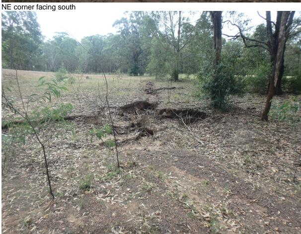
Erosion scour east of dam from run off access road to north, facing north
